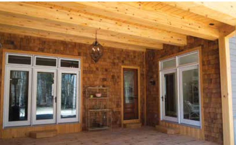
ABOVE: A knotty pine ceiling, black locust floors and cedar shakes give the veranda a rustic feel.
